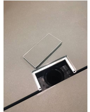
Line Drain Detail
